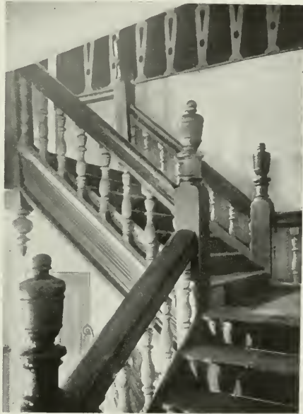
151. Staircase, Boleyn Castle.
